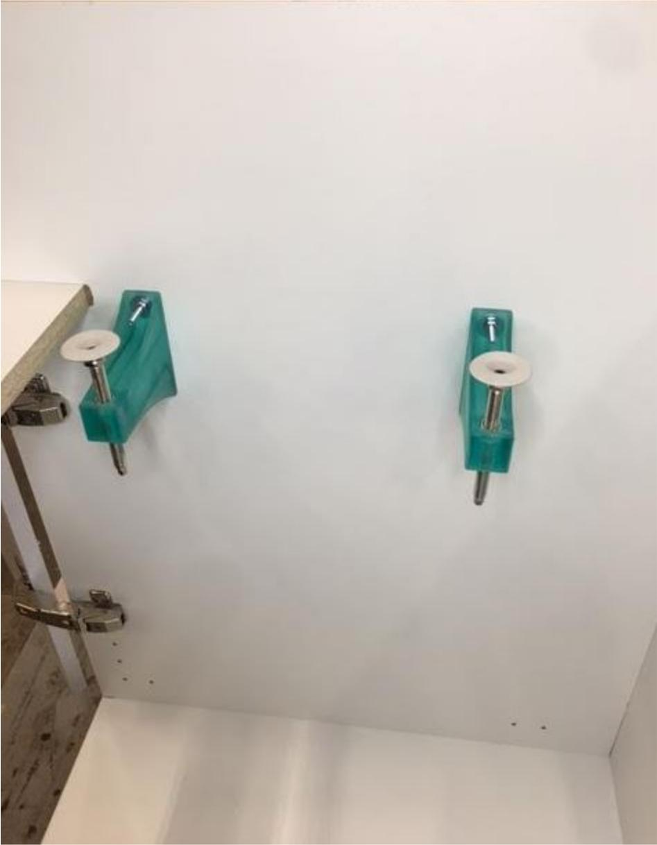
**Making sure all four brackets are fastened securely, install sink and adjust sink to level.**
